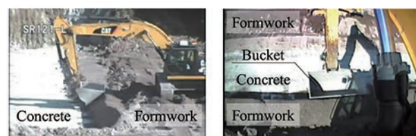
(a) Sight of external camera (b) Sight of cabin camera Fig. 2 Presentation of camera images to the construction machine operator
